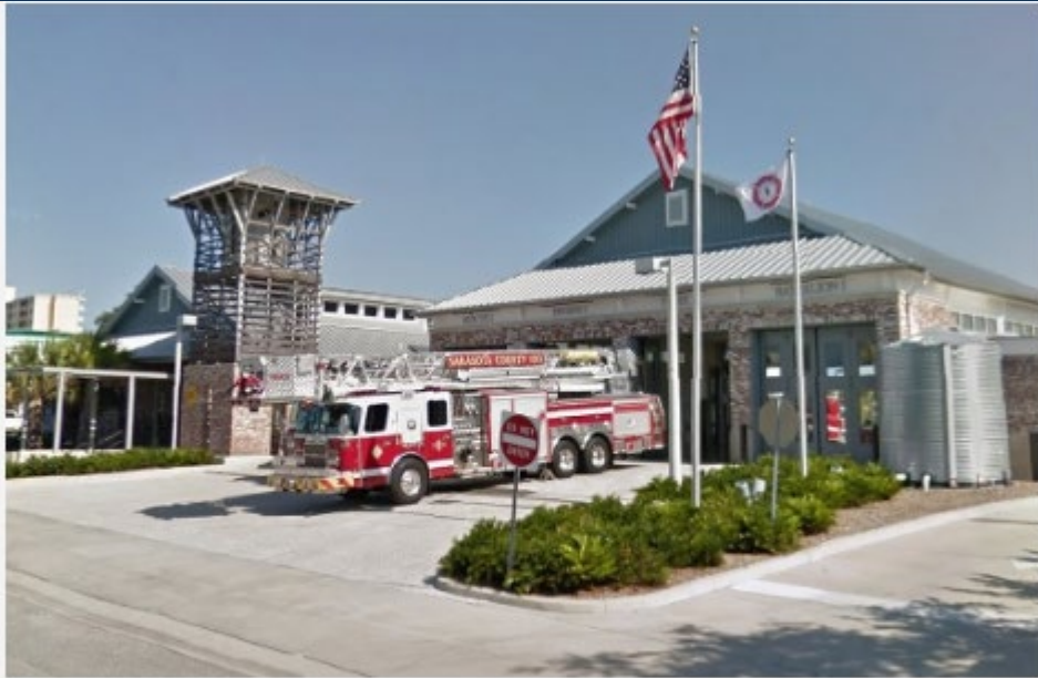
Two cisterns are visible in this photo. The one on the left is located in the tower.
