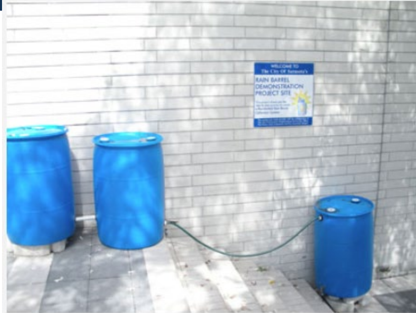
Interconnected rain barrels collect water from the roof of Sarasota City Hall. Water from decorated rain barrels is used to irrigate nearby flowerbeds.
