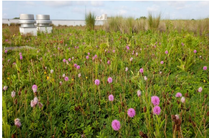
Figure 13 Powderpuff mimosa groundcover on green roof at Escambia County Office Complex (Source: https://gsiphotosflorida.org/ )
