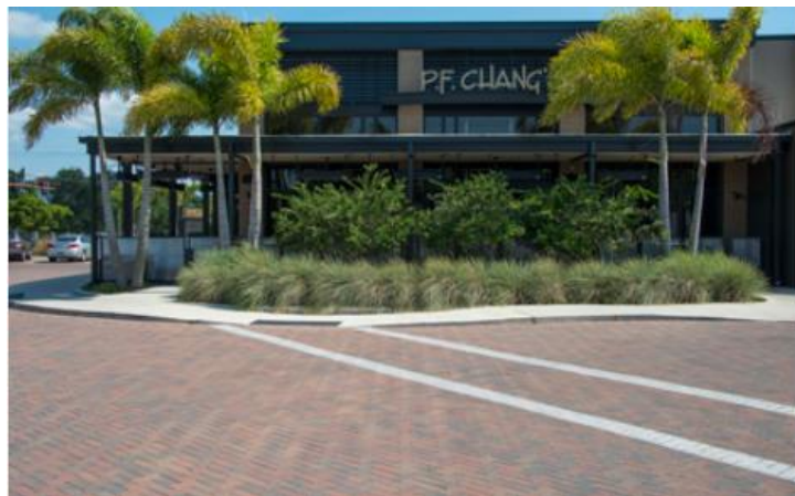
Figure 2 Rain garden and pervious pavers at P.F. Chang's avoided need for retention pond (Source: Sarasota County Government)
